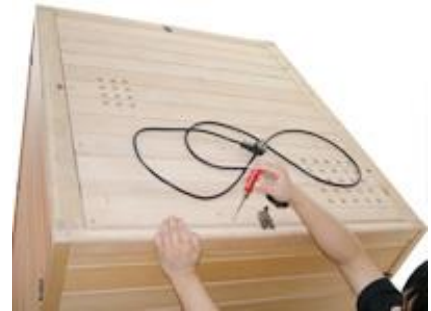
FIG-18 Screw down the Roof Cover
